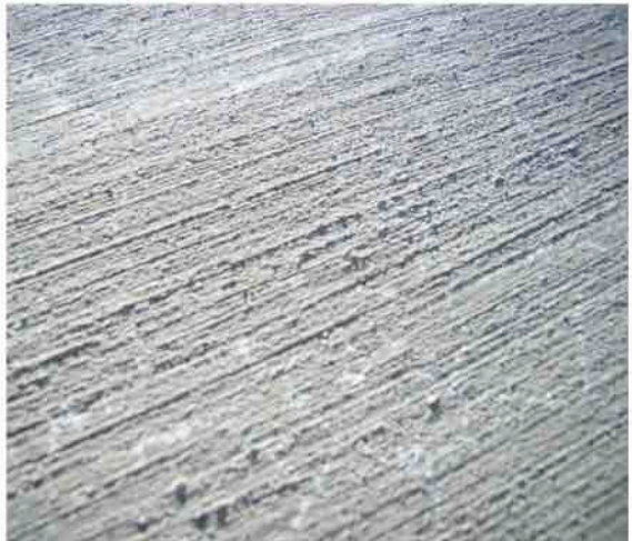
BROOM FINISH CONCRETE
